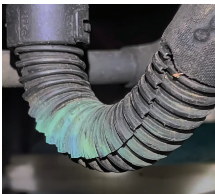
A closer view of the corrosion
