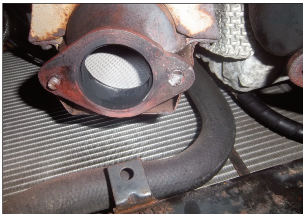
Once the studs had sheared off they needed to be drilled out
